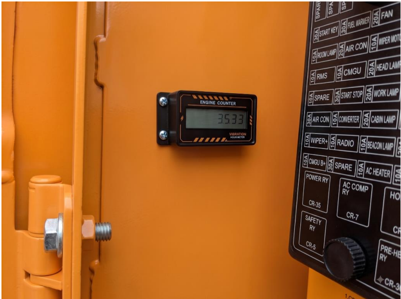
Compact installation near a visible, vibration-active equipment area.
